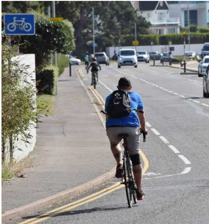
Many of the cycle lanes in BCP are disjointed and fall below current design standards as they are not suitable for users of all ages and abilities and do not provide physical separation from motor traffic, such as these advisory cycle lanes on Shore Road in Poole.
