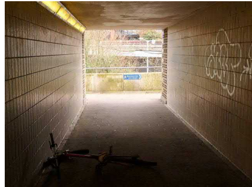
Subway – Richmond Hill, Bournemouth
