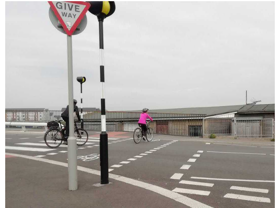
There are several different types of crossings, some of which are designed to accommodate cyclists as well as pedestrians – like this Parallel Zebra crossing in Poole
