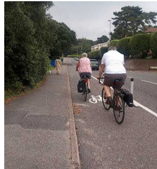
This light-segregated cycle lane, with reflective wands, helps protect people cycling uphill on this busy road in Poole
