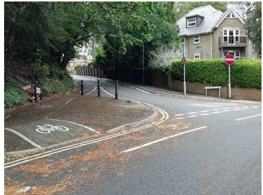
This narrow road in Parkstone was made one-way, but a simple contraflow cycle lane has been included to maintain a direct route for people cycling.
