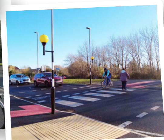
A new parallel crossing on Wimborne Road West
